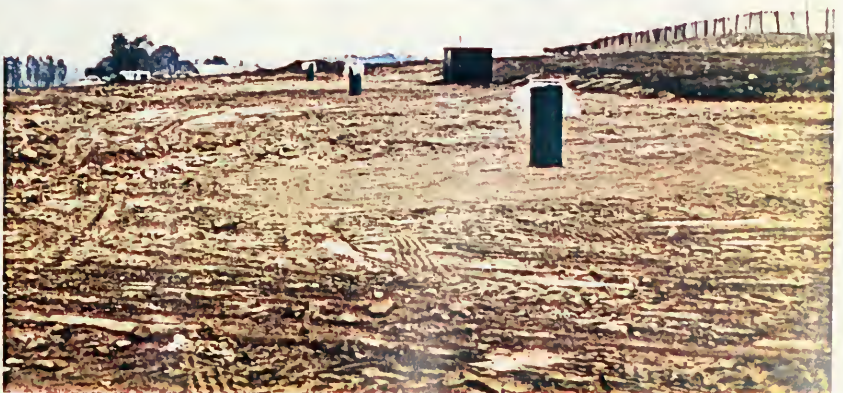
A23: COMPLETED CONSTRUCTION, (GUELPH)
